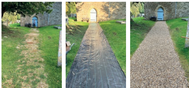
Pictured: the path at the Old Church has been relaid with weed-suppressant matting and new gravel
